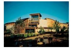
This pavilion consists of two linked buildings, an IMAX theater building and a "Rite of Passage" building. The complex is designed to blend into its surroundings, and utilizes passive solar design with operable windows to facilitate natural cross ventilation. **Location:**
