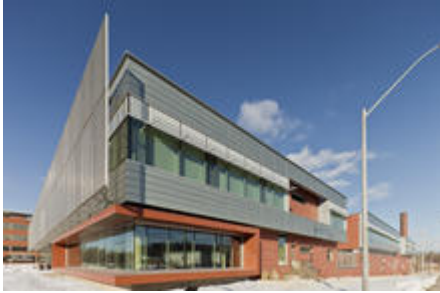
West Facade with Solar Shading - Photo Credit: Peter A. Sellar
